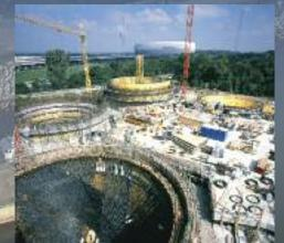
Silos, Shurovo Cement factory, Russia The Shurovo Cement works in Russia had two clinker silos and a raw meal silo, all constructed using European approved CONA CMI technology.
