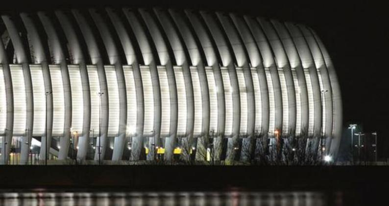
**Europark Shopping Centre, Salzburg, Austria** Internal unbonded CONA CMM PT design delivered excellent static behaviour of the slab and saved valuable construction time.
